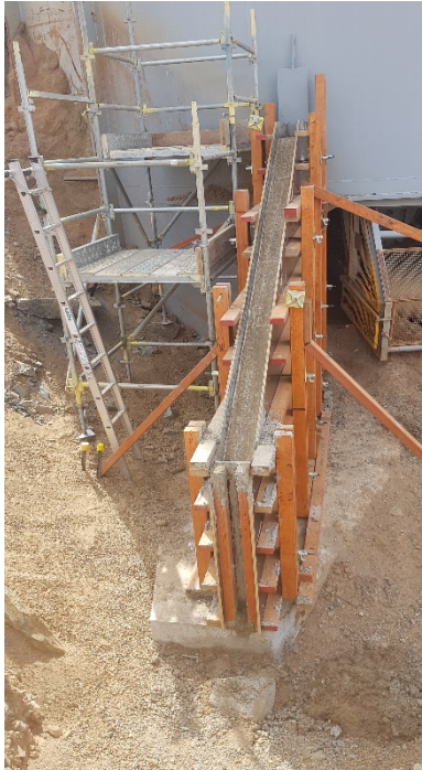
New Secondary Feed Hopper Wing Wall
