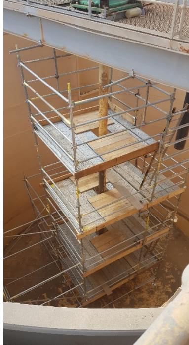
Scaffold in Tank to Refurbish Agitator
